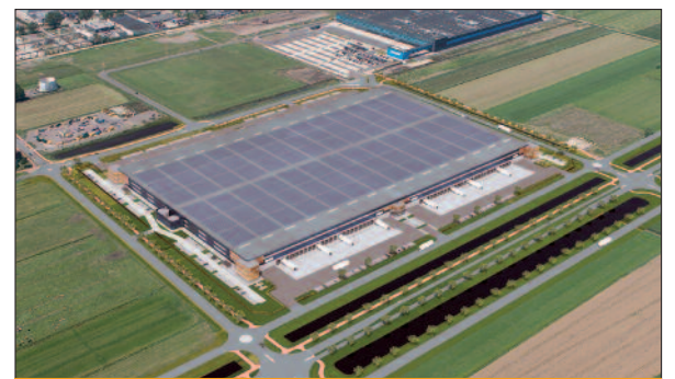
TH MODERN LOGISTIEK COMPLEX DISTRIPORT WAALWIJK
