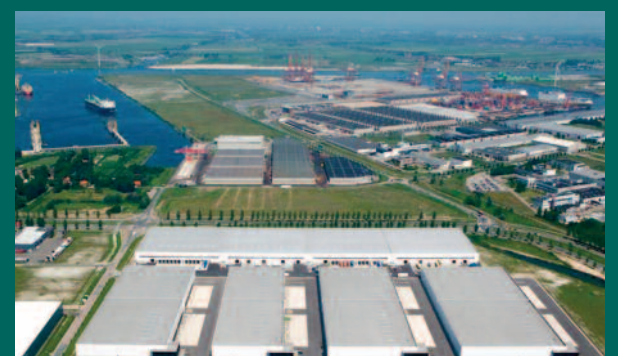
TH SOMERSET FLEXIBELE LOGISTIEKE UNITS OP LOGISTICS PARK UTRECHT
